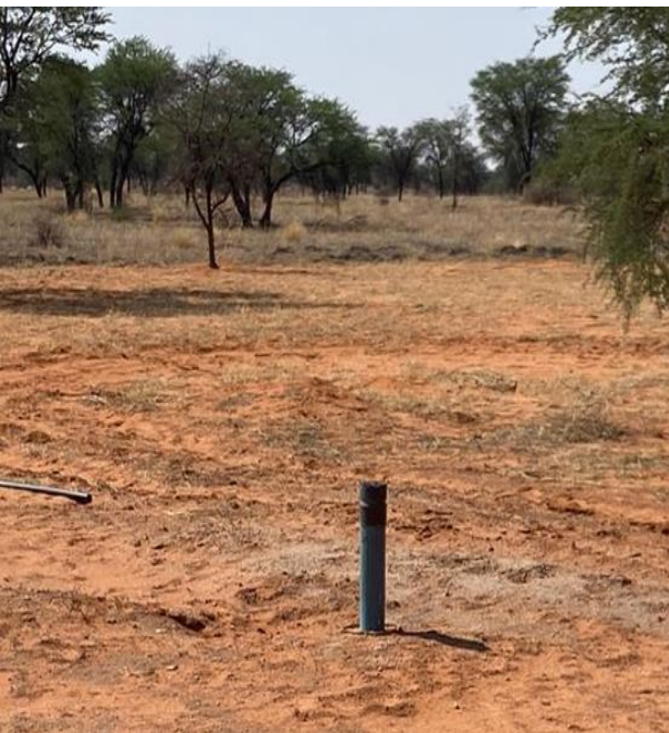
Figure 7: Example of an injection well
